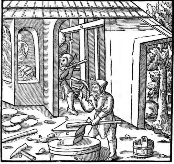
A-POINTED BAR. B-THIN COPPER LAYER. C-ANVIL. D-HAMMER.
